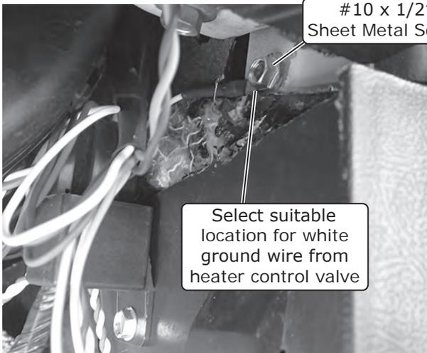
Select suitable location for white ground wire from heater control valve
