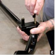
3. Slide the billet mount over the bushing, then the two bolts, then the mounting plate, then the two bolt spacers (Photo C).
